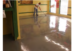
Commercial grade 3-coat random flake system for a local bike shop.
