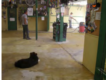
Commercial grade 3-coat random flake system for a local bike shop.
